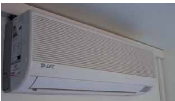
air-conditioning system: inner part
